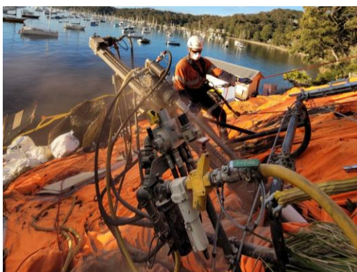
Slope Stabilisation at Clareville Beach
