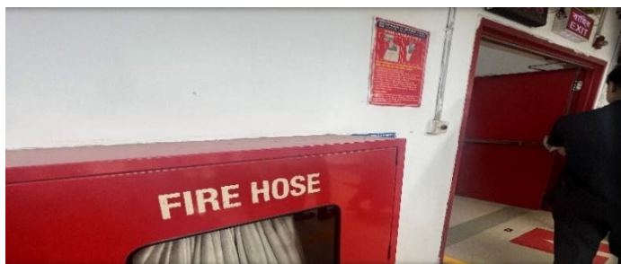
Fire and structural safety have improved since the Rana Plaza collapse | Natural Denim, Dhaka
